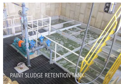
PAINT SLUDGE SYSTEM PUMPS
