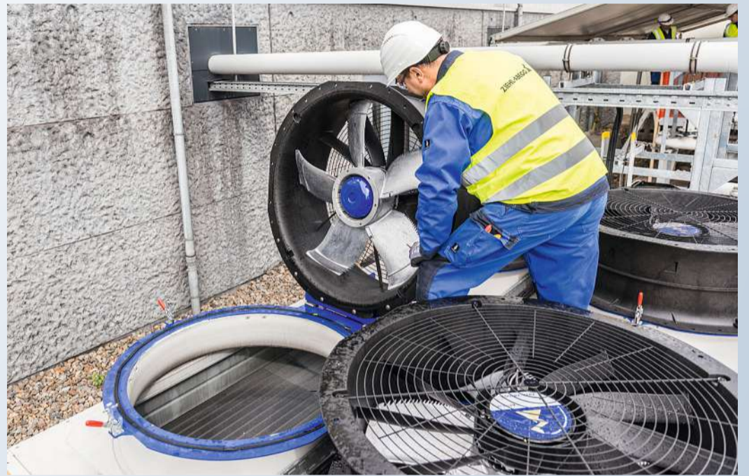
For their client BritNed in Maasvlakte, Netherlands, ZIEHL-ABEGG replaced the fans that cool the converter stations. BritNed is the operator of the high-voltage direct-current cable system that connects Great Britain and the Netherlands via marine power cables. The new fans enable BritNed to reduce their electricity consumption and lower their CO 2 emissions.
