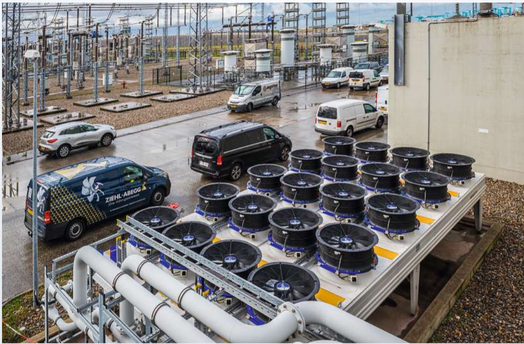
For their client BritNed in Maasvlakte, Netherlands, ZIEHL-ABEGG replaced the fans that cool the converter stations. BritNed is the operator of the high-voltage direct-current cable system that connects Great Britain and the Netherlands via marine power cables. The new fans enable BritNed to reduce their electricity consumption and lower their CO 2 emissions.
